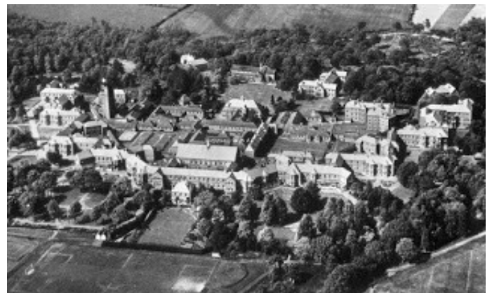
AIR VIEW OF HELLINGLY HOSPITAL, HAILSHAM, SUSSEX.
